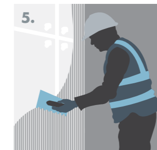
5. Applying notches within the basecoat.
