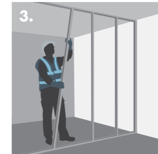
3. Twisting Knauf Acoustic 'C' Studs into position.
