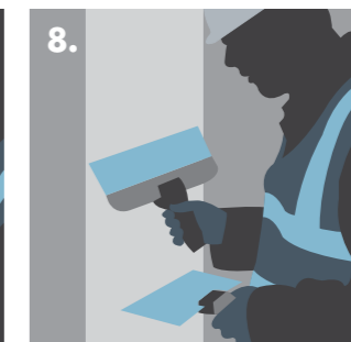
8. Tape and joint for a seamless finish.
