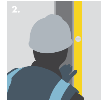
2. Fixing Knauf 'U' Channel to form the partition frame.
