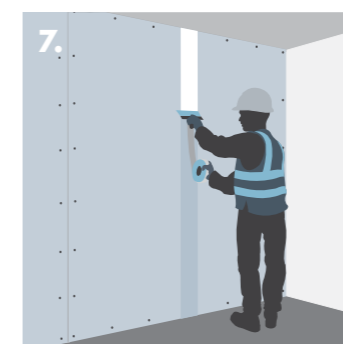
7. Taping and jointing for a seamless finish.
