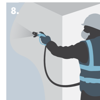
8. Finishing using Knauf plaster.
