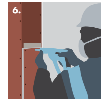
6. Fixing outer layer of Knauf Fire Panel.
