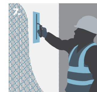
7. Covering mesh with basecoat.
