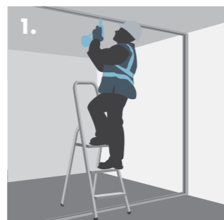
1. Fixing the head track.
