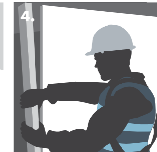
4. Positioning Knauf 'C-T' Stud to lock Knauf Core Board into place.
